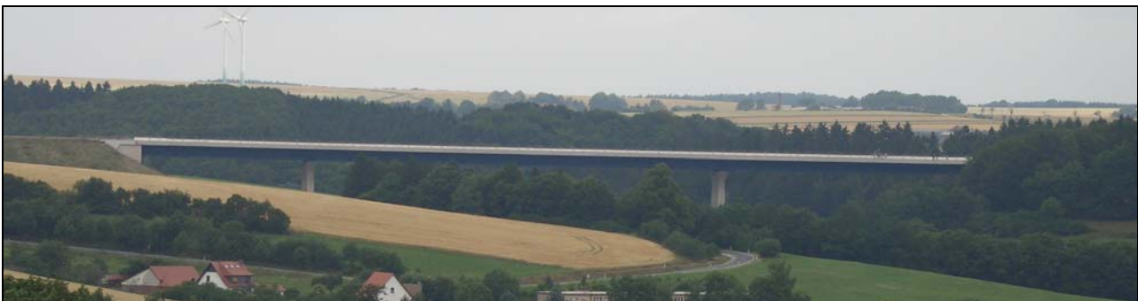
Fig. 1. The Steinbachtal Bridge on the Southharz Autobahn (A38) near Bodenrode, Thuringia, Germany.
